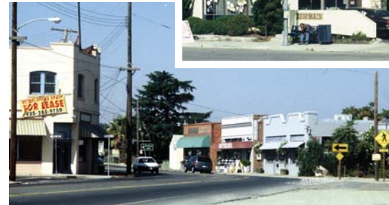
Buildings and street frontages in Oakley do not create an attractive downtown today.
